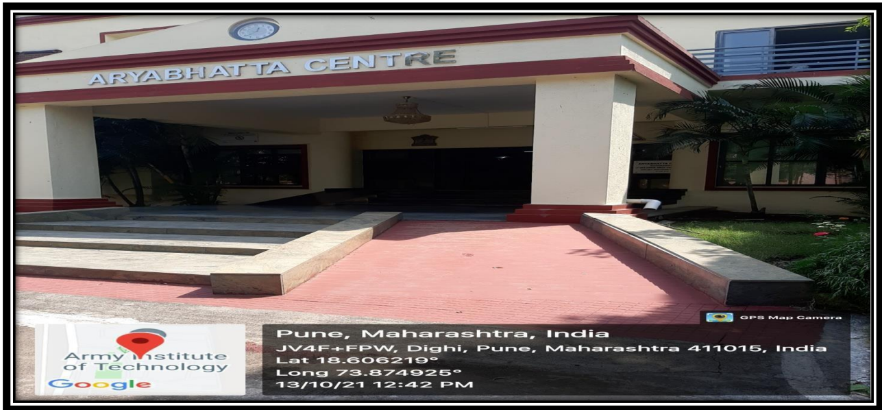
Ramp in Campus
