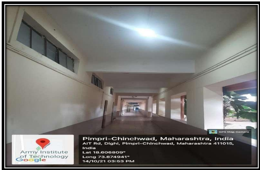
Corridor LED Lights
