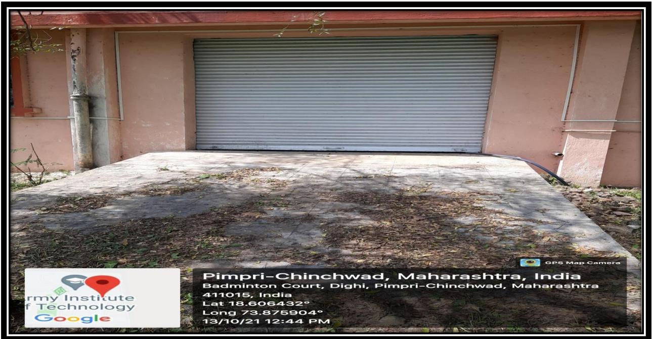
Ramp in Campus
