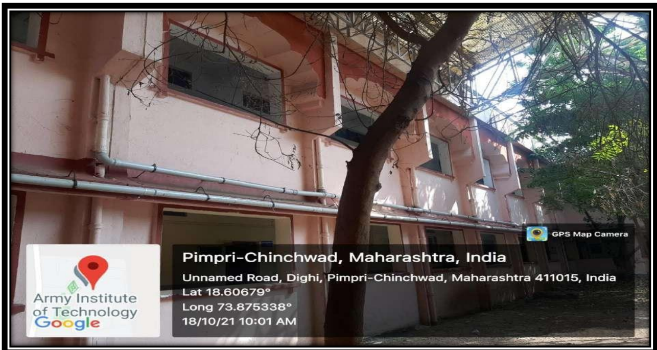
STORM DRAINAGE PIPE SYSTEM FOR RAIN WATER HARVESTING
