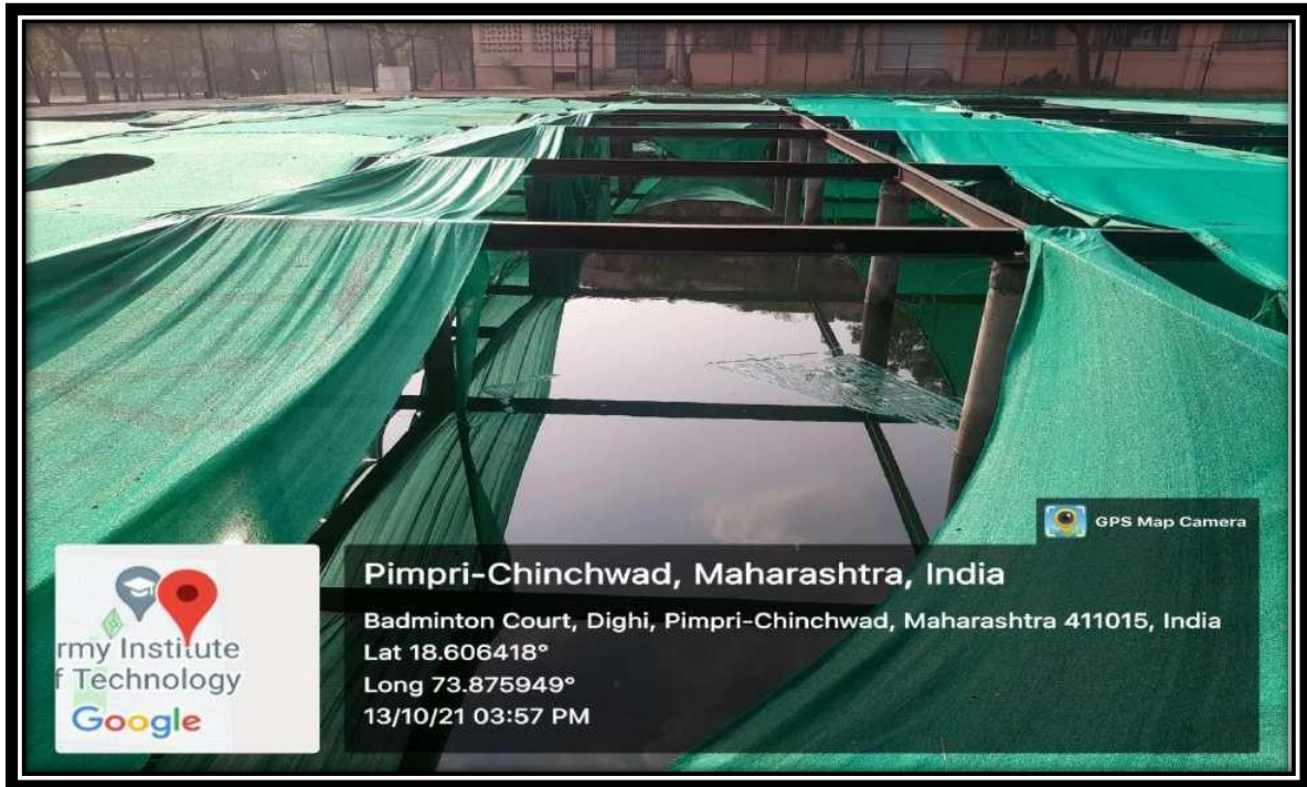
Rain Water Storage Tank
