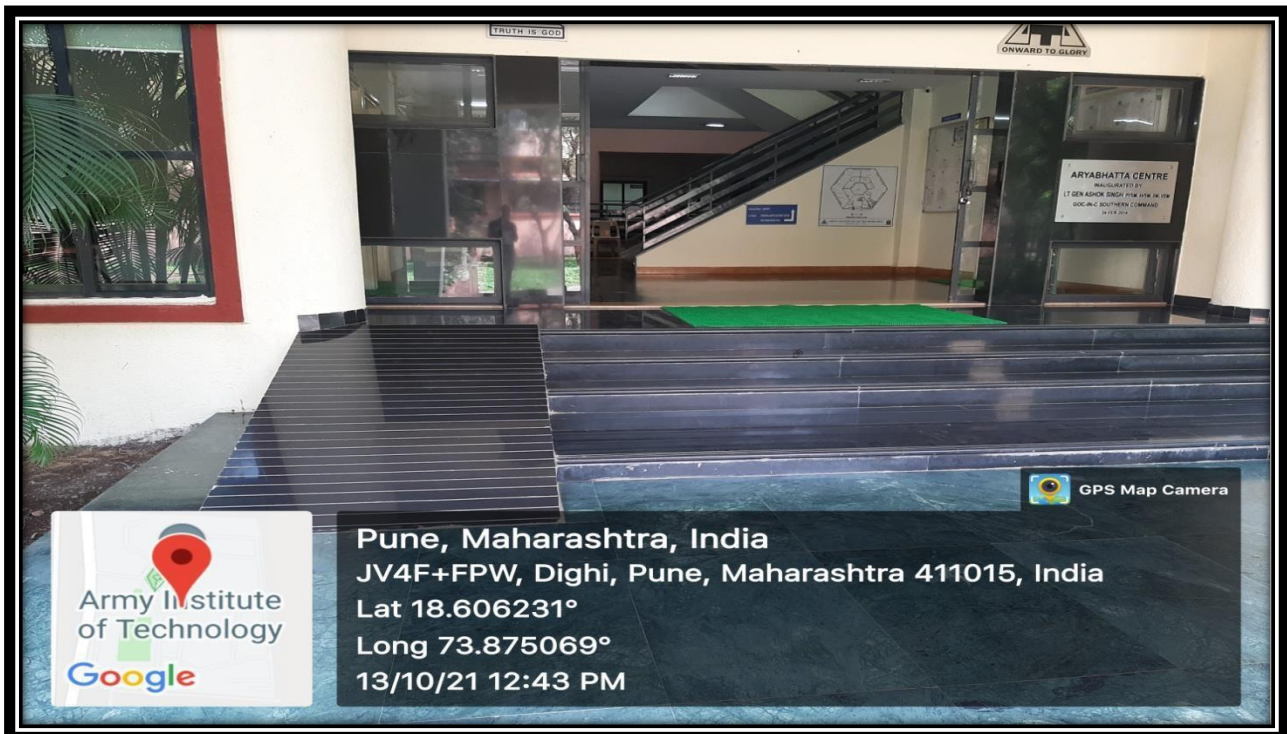
Ramp in Campus
