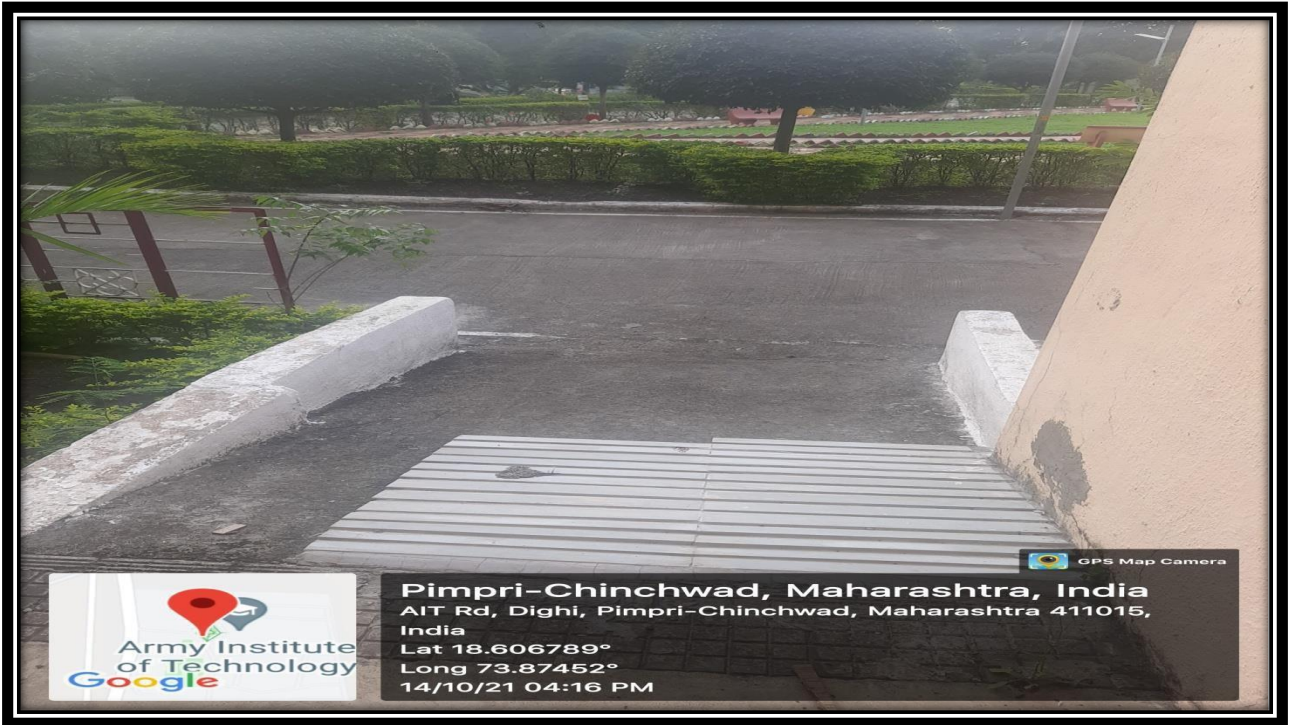
Ramp in Campus
