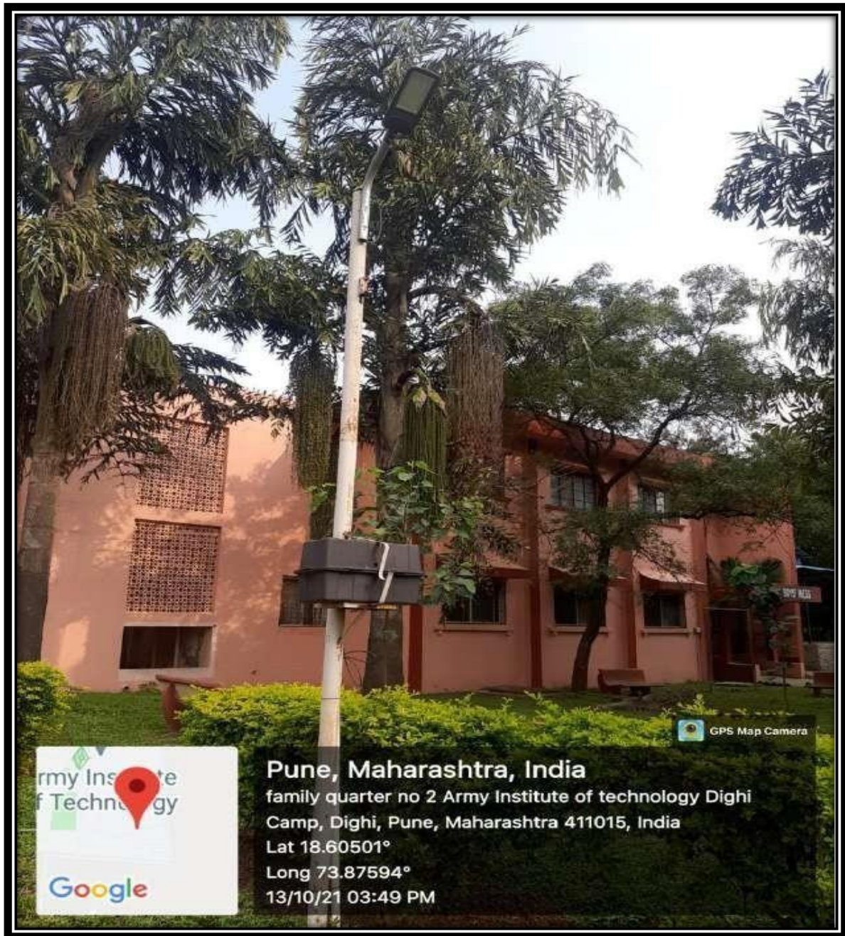
Use of LED Bulb Led Street Light
