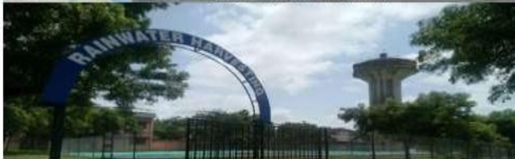
Construction of tanks and bunds
