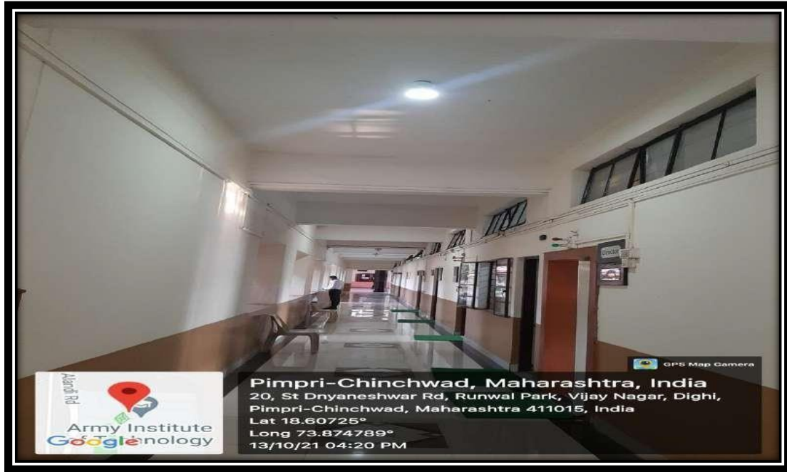
Corridor LED Lights
